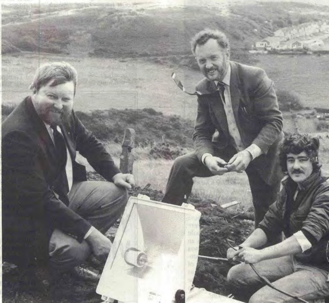
Working on the floodlighting installation we see, from left to right : engineers Allen Carr and Clive Wintle, with craftsman electrician Colin Appleton.
