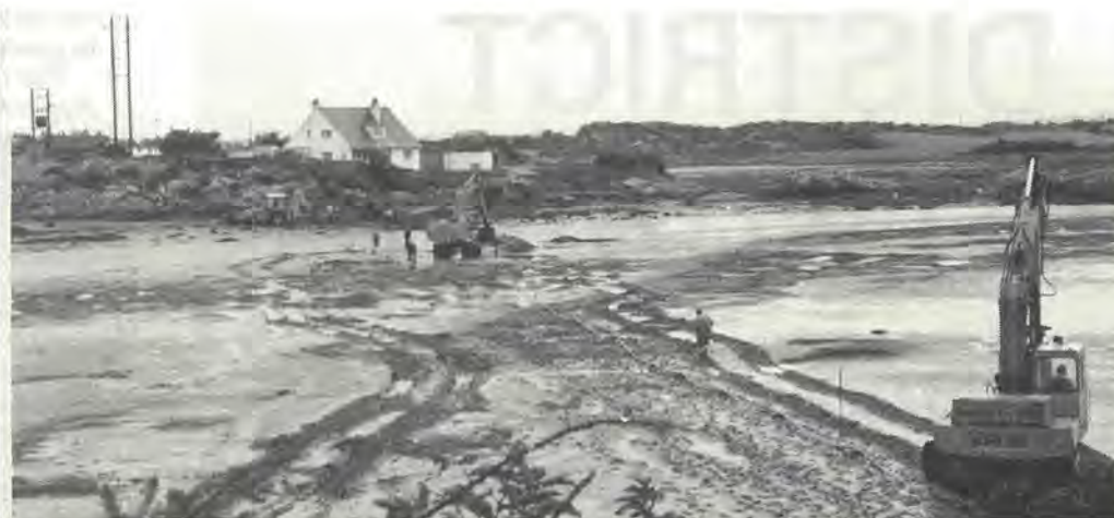
Hymac excavators busily digging the trench across the estuary in readiness for the submarine cable. In the left distance is the extra-high, now redundant, 'H' pole which was used to carry the line over the water. The normal height pole, with its transformer, is positioned ready for its new connection.
